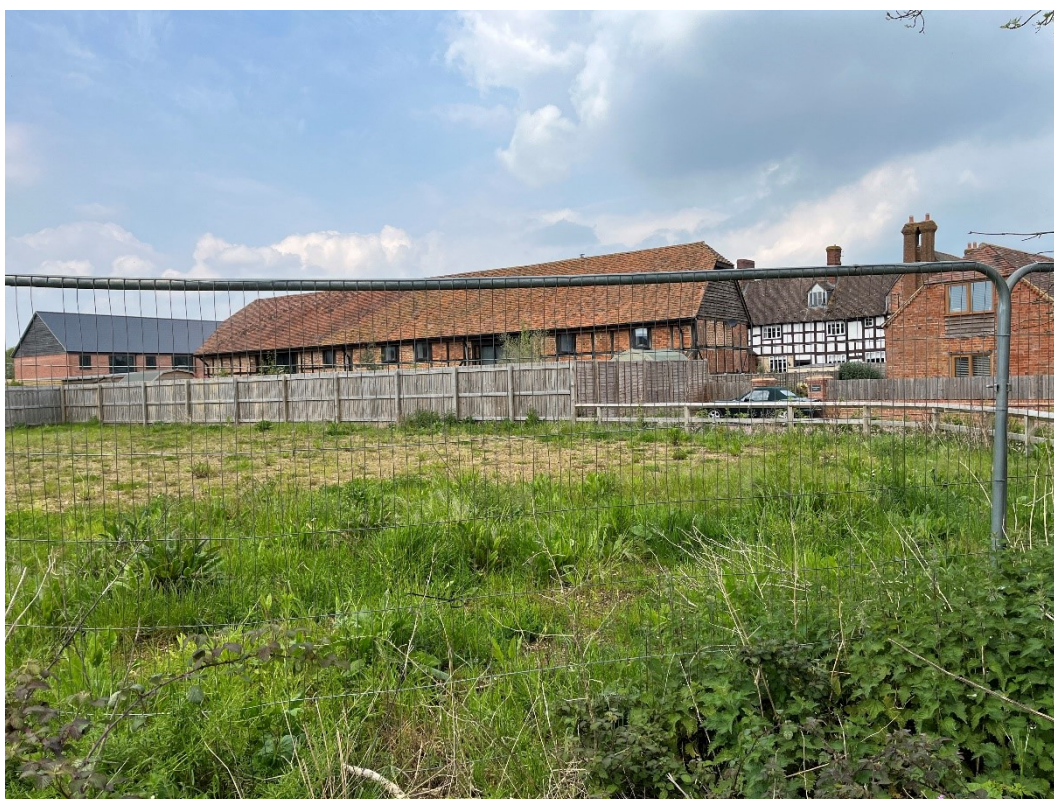
Figure 19: View of the Barn (front) and rear range of Allesborough Farmhouse (back) from Rebecca Road
