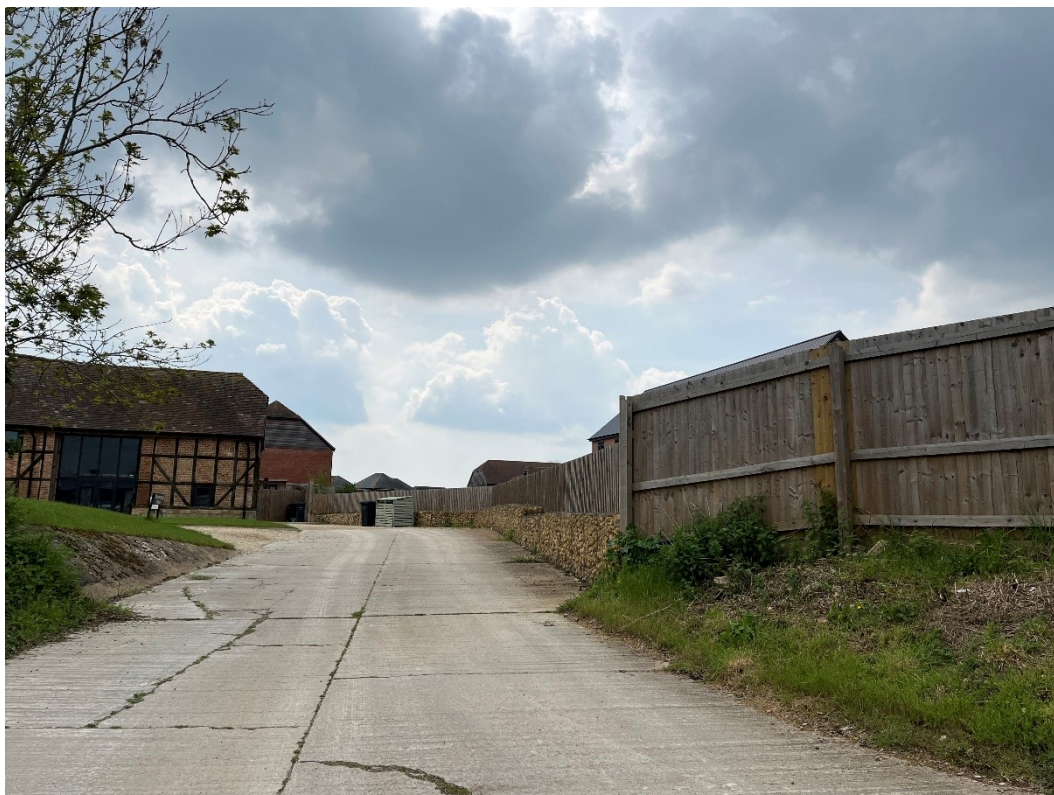
Figure 16: View west towards the Site from the B4084
